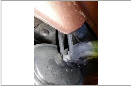
Check exhaust system condition 14060 - Image 1 of 2
