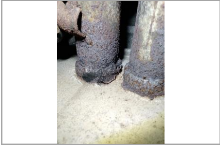
Check exhaust system condition 14060 - Image 1 of 2
