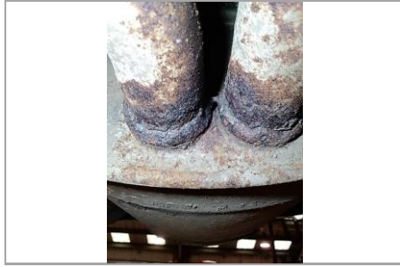
Check exhaust system condition 14060 - Image 2 of 2
