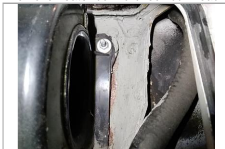
Remove heater box lid-check bulkhead
