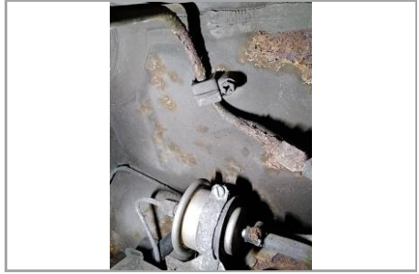
Check fuel pump pipes/filter package 47045 - Image 2 of 2
